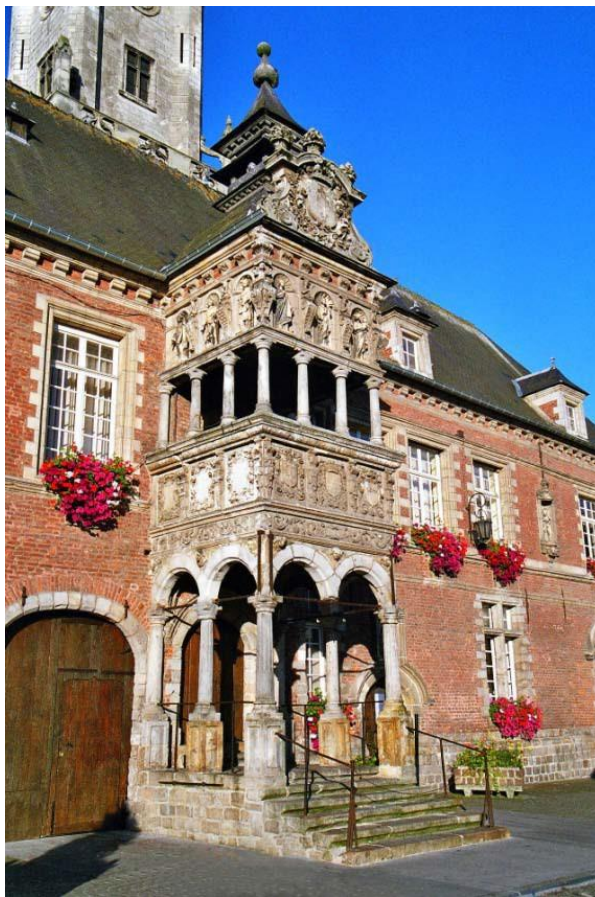
Detailed view of the Town Hall Main Entrance Hesdin
