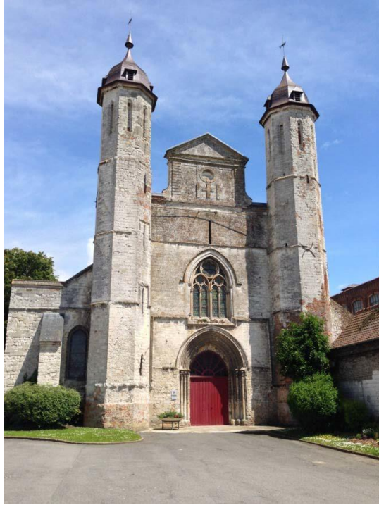
Abbey of St. Georges and St. Silvin, in Auchy-lès-Hesdin. Earliest parts of structure date to 700AD
