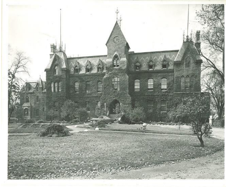
Figure 9. Académie du Plateau, home of the Scientific and Industrial School (Archambault School) (1873-1876) that later became École Polytechnique de Montréal
